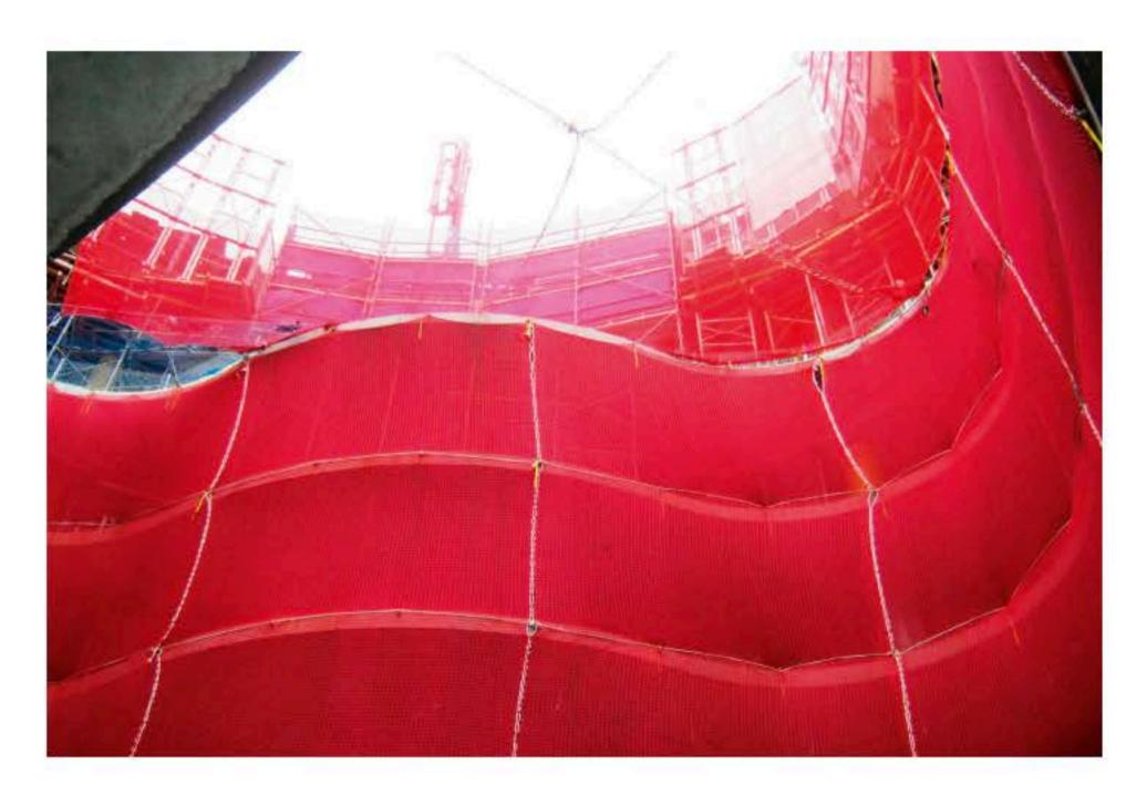
These nets protect completely the voids so that there is no possibility that workers could fall into the void from the inside. In addition to protecting the holes in the floor, they also serve to prevent the fall of people from open windows and stairs.
