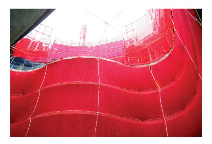
These nets protect completely the voids so that there is no possibility that workers could fall into the void from the inside. In addition to protecting the holes in the floor, they also serve to prevent the fall of people from open windows and stairs.
